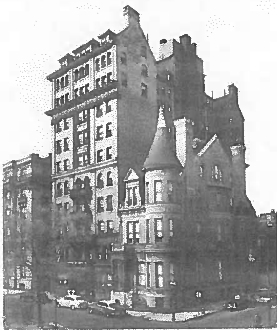
George Graham house, southwest corner of Washington Place and Madison Street, designed by George Archer, 1888, and behind it, the Stafford Hotel, designed by Charles E. Cassell, 1893. Peale Collection, Maryland Historical Society
